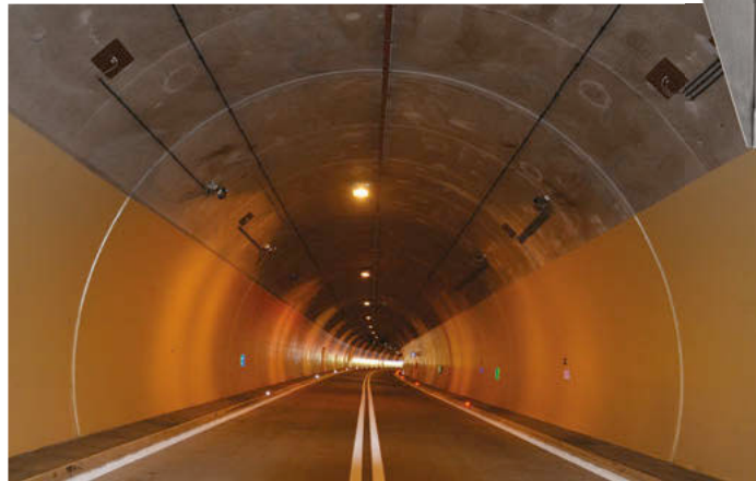
Above: Luminance meters adapt lighting in tunnels to their surroundings. For example, to daylight or dark at the entrance/exit
